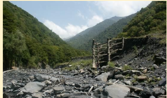
Protective dam destroyed by debris flows. Duruji River upstream of Kvareli town
