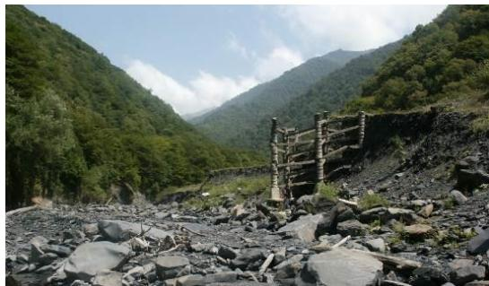
Protective dam destroyed by debris flows.
