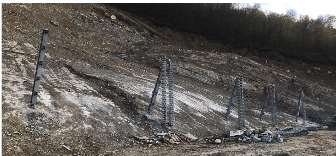
Fig. 7. Ongoing construction in April 2018 of posts for rock fall barrier by Trumer protecting the Samadlo road. Photo: D. Dumbadze
