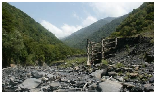
Protective dam destroyed by debris flows. Duruji River upstream of Kvareli town
