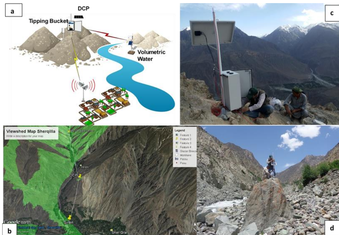
Fig. 6. a) Describes the early warning system and its components i.e. water content sensor, data collection platform, tipping bucket and siren system. b) Selection of site through the remote sensing to view the line of site for EWS. c) AKAH staff installing DCP at the identified site. d) Installation of water content sensor by staff. Photo Credit AKAH Pakistan
