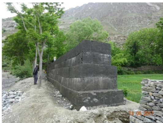
Fig. 11. Cross-sectional view of protection wall along the gorge at the convex portion of the meandering stream
