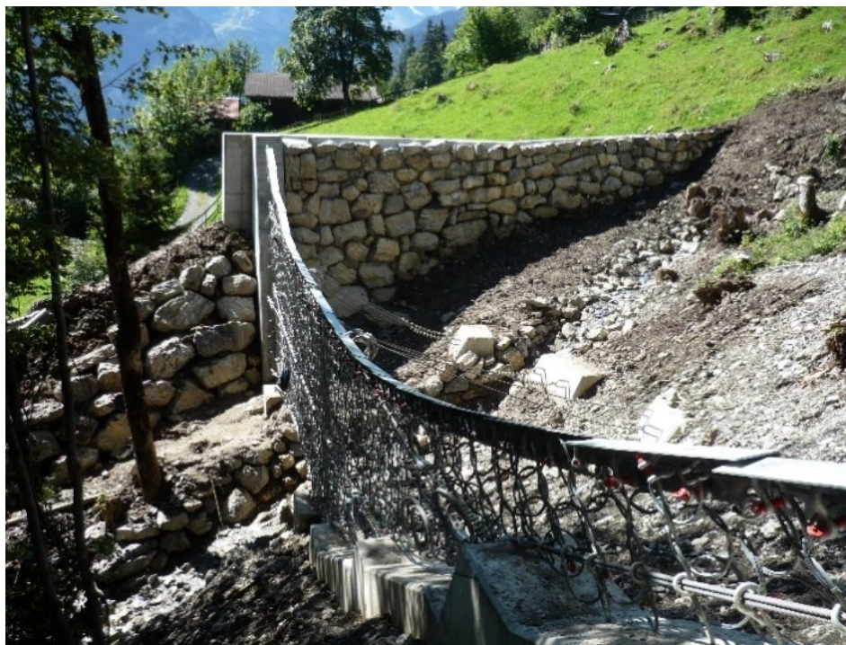
Fig. 9. Debris flow barrier in Isenflue above a settlement. The outer bank of the stream was reinforced with a rock wall
