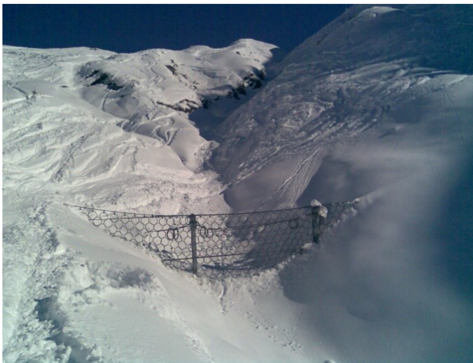
Fig. 4. same net than in Fig. 3, partially snowed in during winter. The snow load has to be taken into account when designing the barrier
