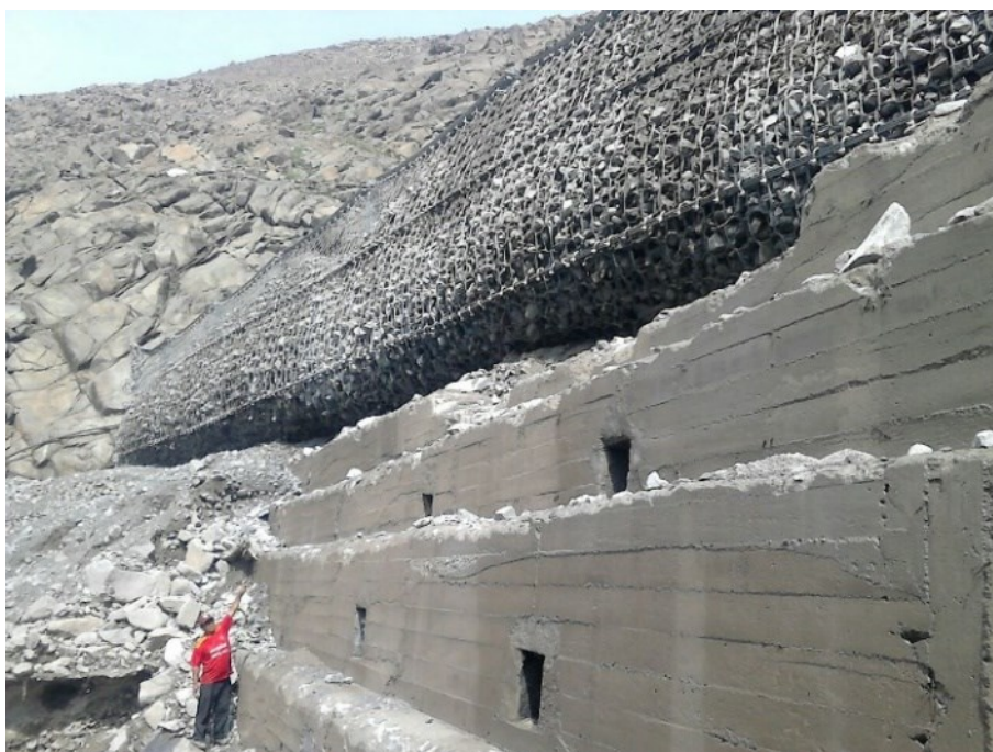
Fig. 11. Filled debris flow barrier in 2017 in Peru, protecting successfully a large city downstream
