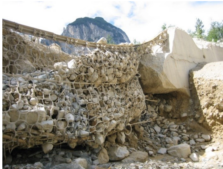
Fig. 5. Washed out anchoring of the debris flow barrier number 25 in the Illgraben channel. Anchoring partially in loose material and partially in disused concrete debris flow barrier
