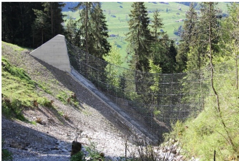
Fig. 12. Special construction of a debris flow barrier in Hüpach, in Switzerland, with a width of 40m and a netting height of 10 m
