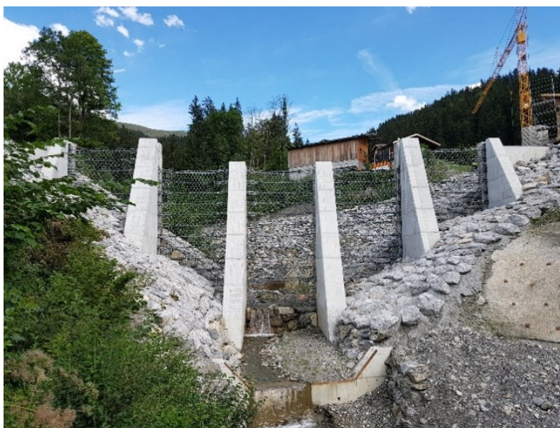
Fig. 13. Another special construction acting as a debris flow barrier in Sitäbach, consisting of concrete slices piled up and netting mounted in between
