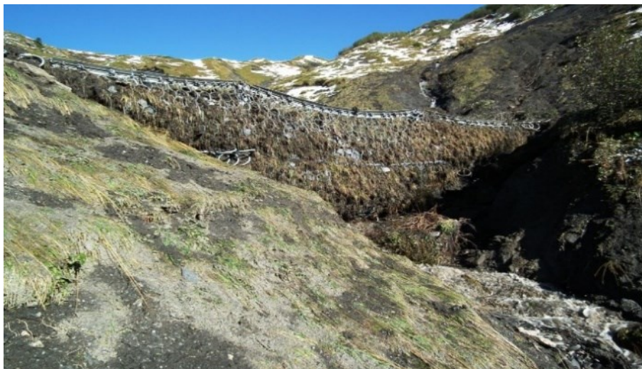
Fig. 10. Debris flow protection barriers, successfully filled in Hasliberg in 2011
