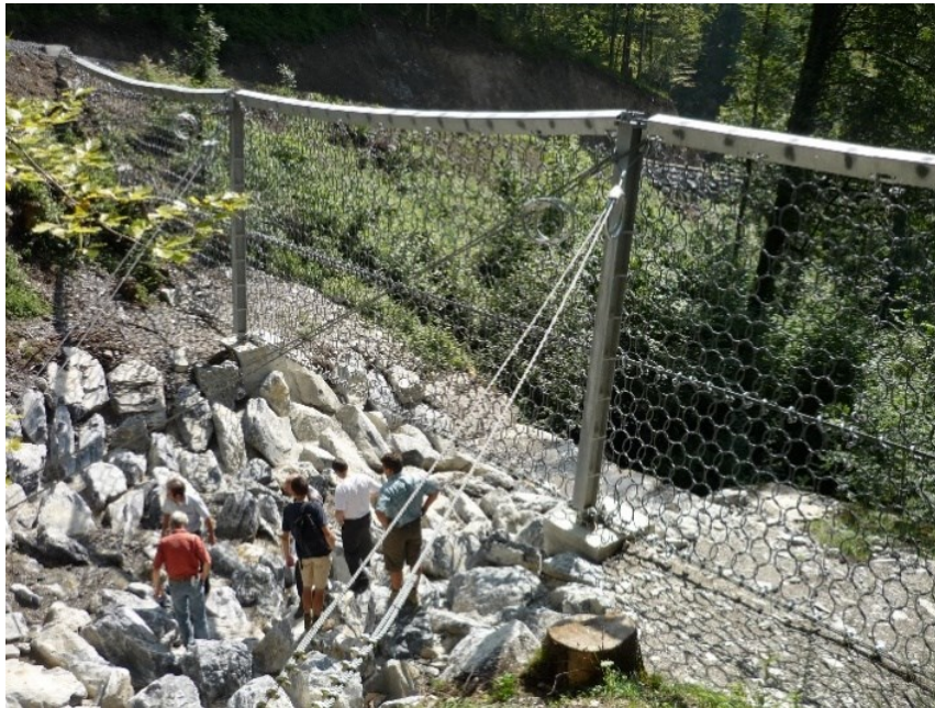
Fig. 2. UX debris flow barrier, with posts for wider stream channels application. Example of the Trachtbach in Switzerland. Additional kolk protection, riprap and lean concrete were placed along the stream bed
