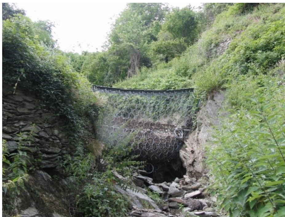
Fig. 8. partially filled debris flow barrier above the German Railway close to Koblenz
