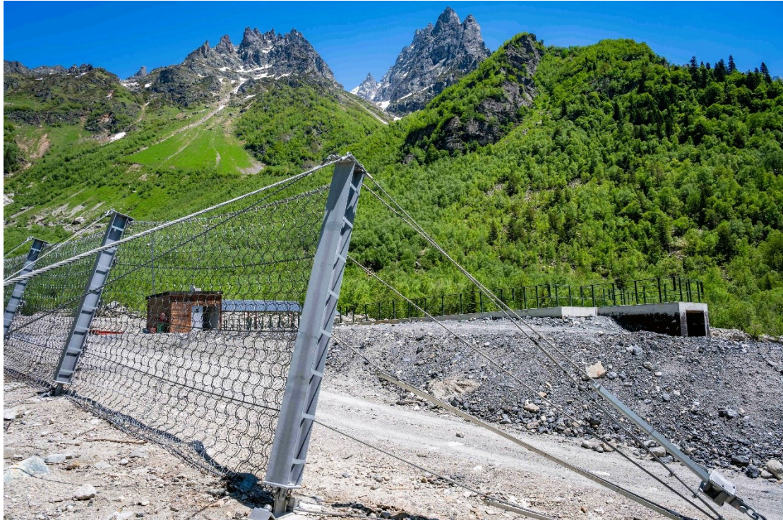
Fig. 5. A Trumer Schutzbauten TSV-2000-ZD H4 hinged rockfall barrier with 8 m post spacing has been installed to protect the new intake building of the Mestiachala HPP
