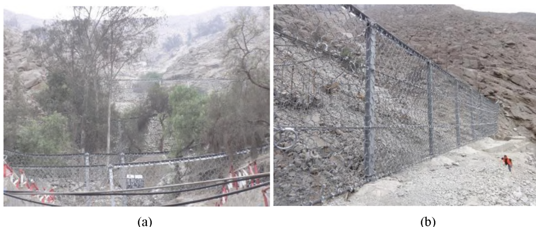
Fig. 8. Multi-level installation of flexible ring net barriers (left). The highest barrier is the largest in South America (right)
