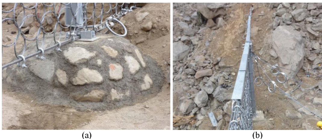
Fig. 6. (a) Scour protection around the posts for UX-barriers; (b) abrasion protection for the top support rope
