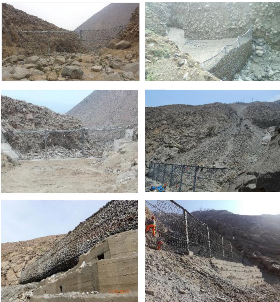
Fig. 9. Before (2016) and after the debris flow event (2017) and subsequent maintenance (2018) for the stream San Pedregal (above) and Carrosio (below)
